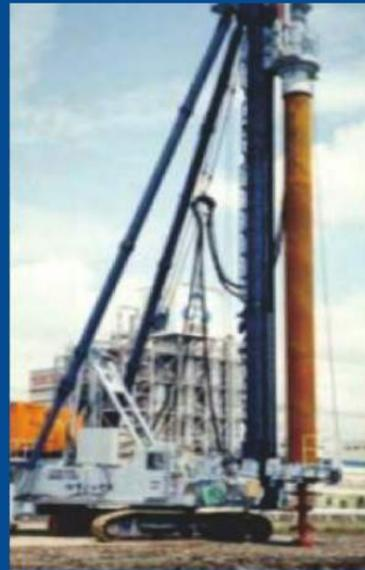
Steel pipe composite pile drilling rig
